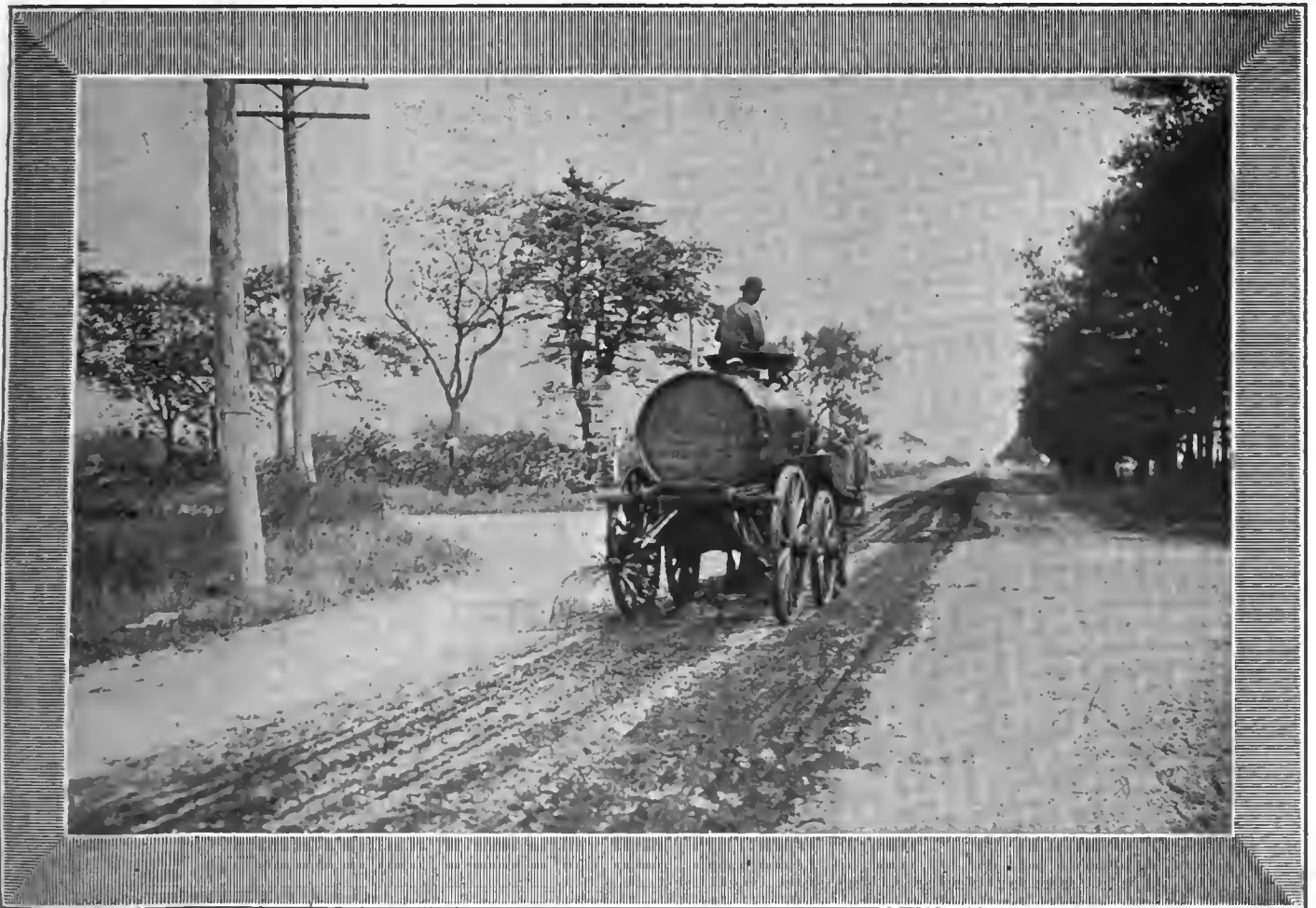
ONE OF THE SPRINKLING CARTS OILING THE VANDERBILT CUP COURSE ON LONG ISLAND WITH CRUDE PETROLEUM.
